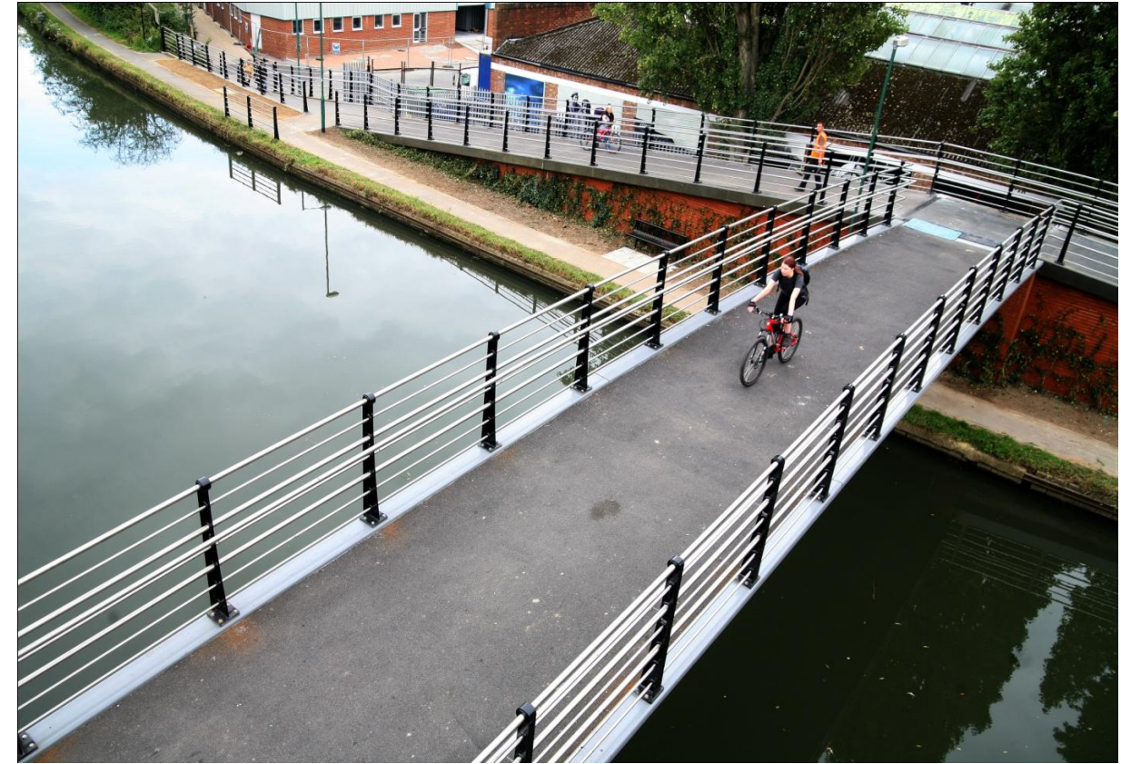
Not only did the new "Grand Union Bridge" facilitate significant improvements for pedestrian and cyclist access to the Grand Union Canal, near Alperton, it was unique in its overarching objectives and aspirations to design out crime.
