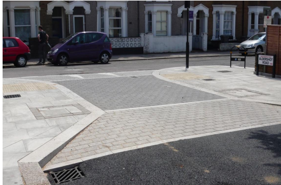
A simple speed reduction intervention. Tightened corner radii coupled with a raised surface and a 'one in-one out' system heightens driver awareness and reduces vehicle speeds. A pedestrian-vehicle collision is likely to have far less severe consequences as a result of this simple, yet effective, measure. Kilburn "Streets for People" project.
